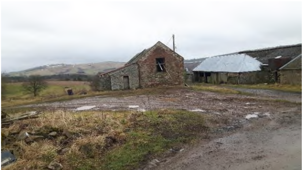
Figure 3.1 Topography of existing site as observed from access road on 16.03.2018
